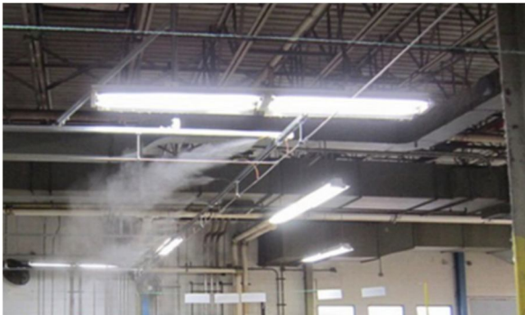
Applications include industrial sites where odor, dust, and humidity control is desired. Misting combined with proper ventilation can provide a high cooling effect.
