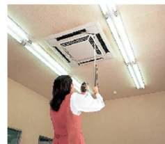
Check airflow rate of air conditioners
