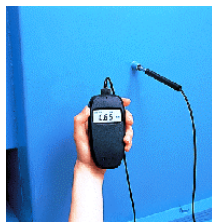
Measuring airflow rate inside ducts
